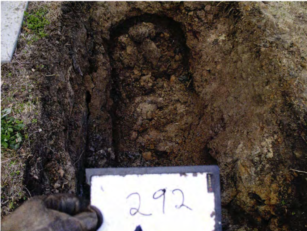
Picture 2: UST 292Birch excavation.
